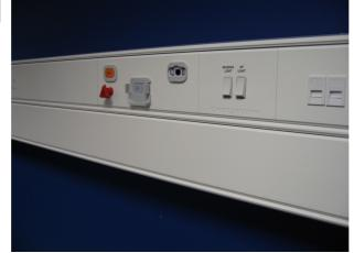
the respective manufacturer's product range. As, with our mains sockets, no screw fixings are visible on the trunking lid.
